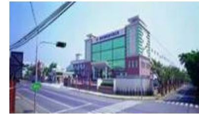
Tsang Yow Chung-Shan plant,TAIWAN(10,710 m 2 )
