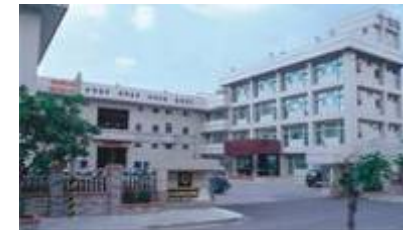
Tsang Yow Cheng-gong plant,TAIWAN(5,200 m 2 )
